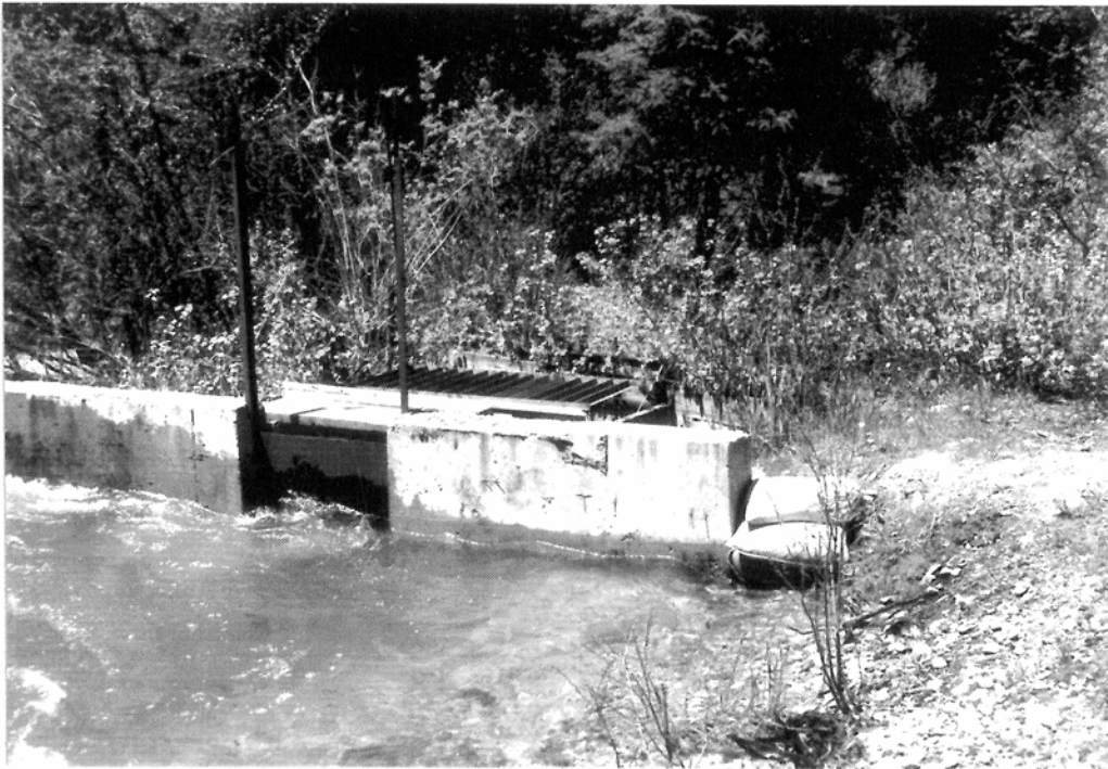
Diversion Dam, Darby Creek
